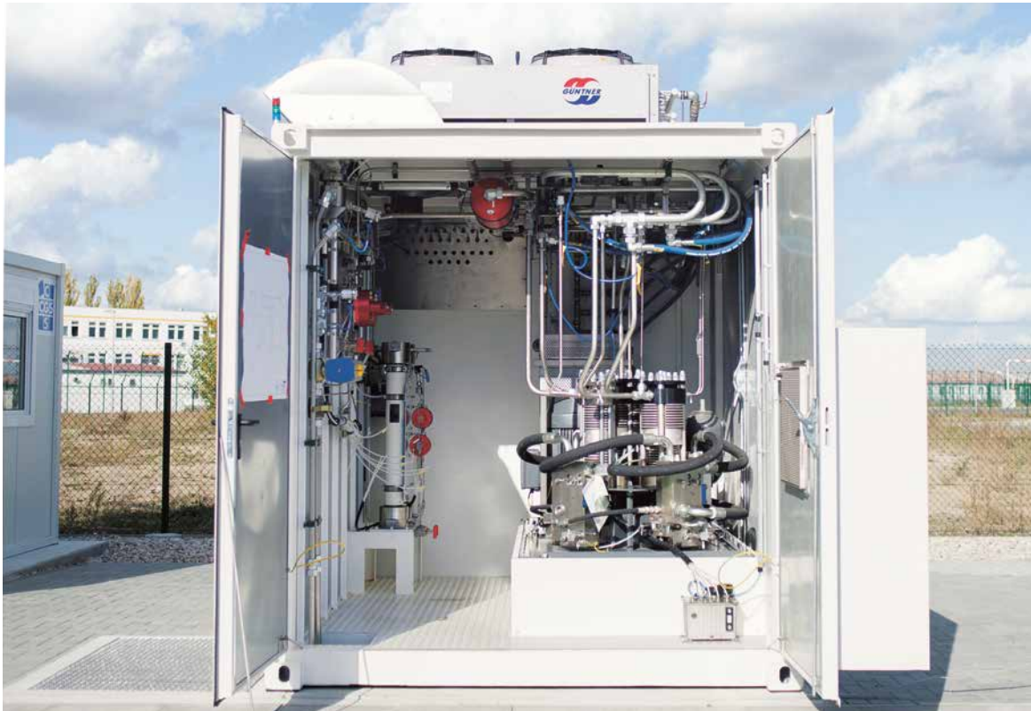
View into a completely assembled hydrogen compressor station.
